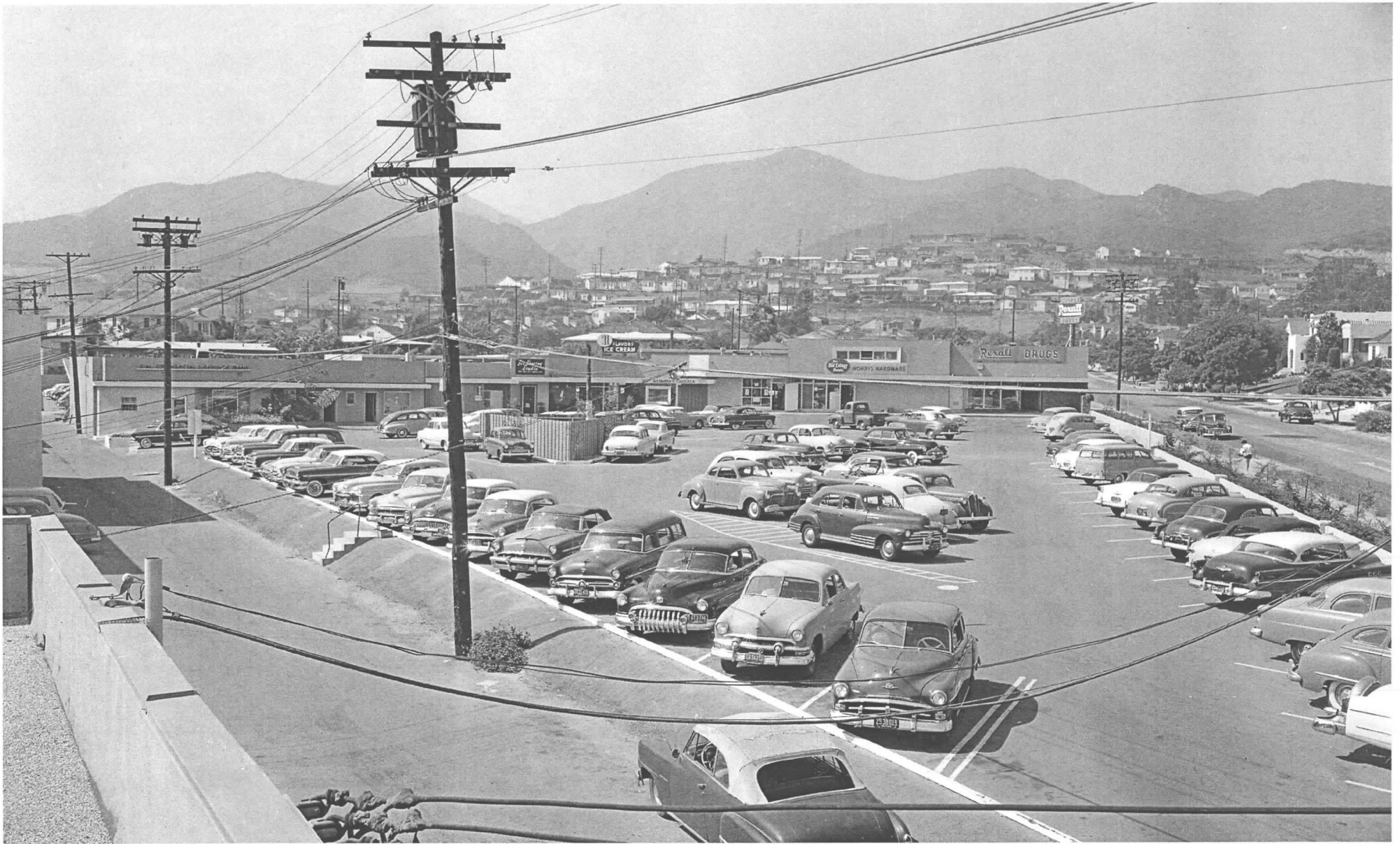
Swarthmore and Monument after Completion of Parking Lot August 1954.
