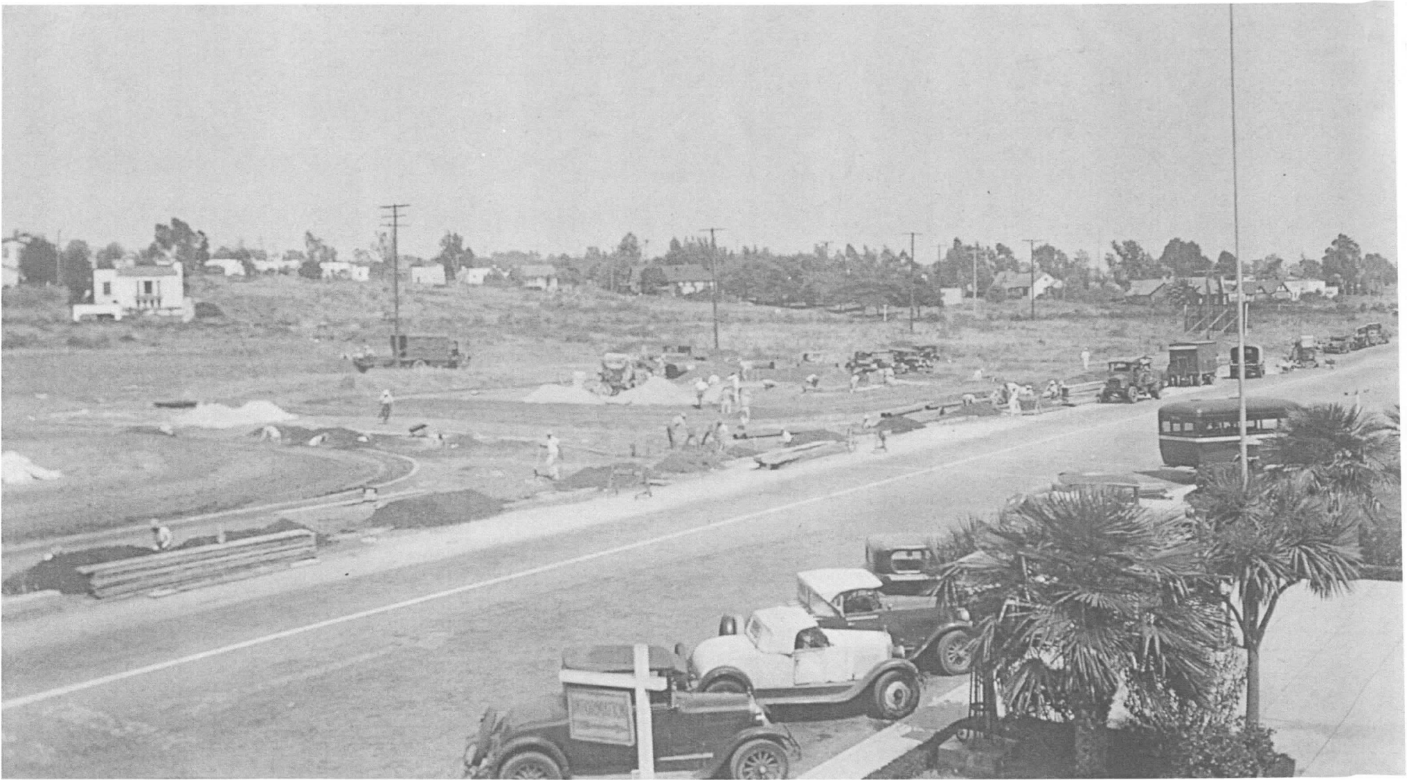
The Building of the Entrance to North Swarthmore Circa 1935
