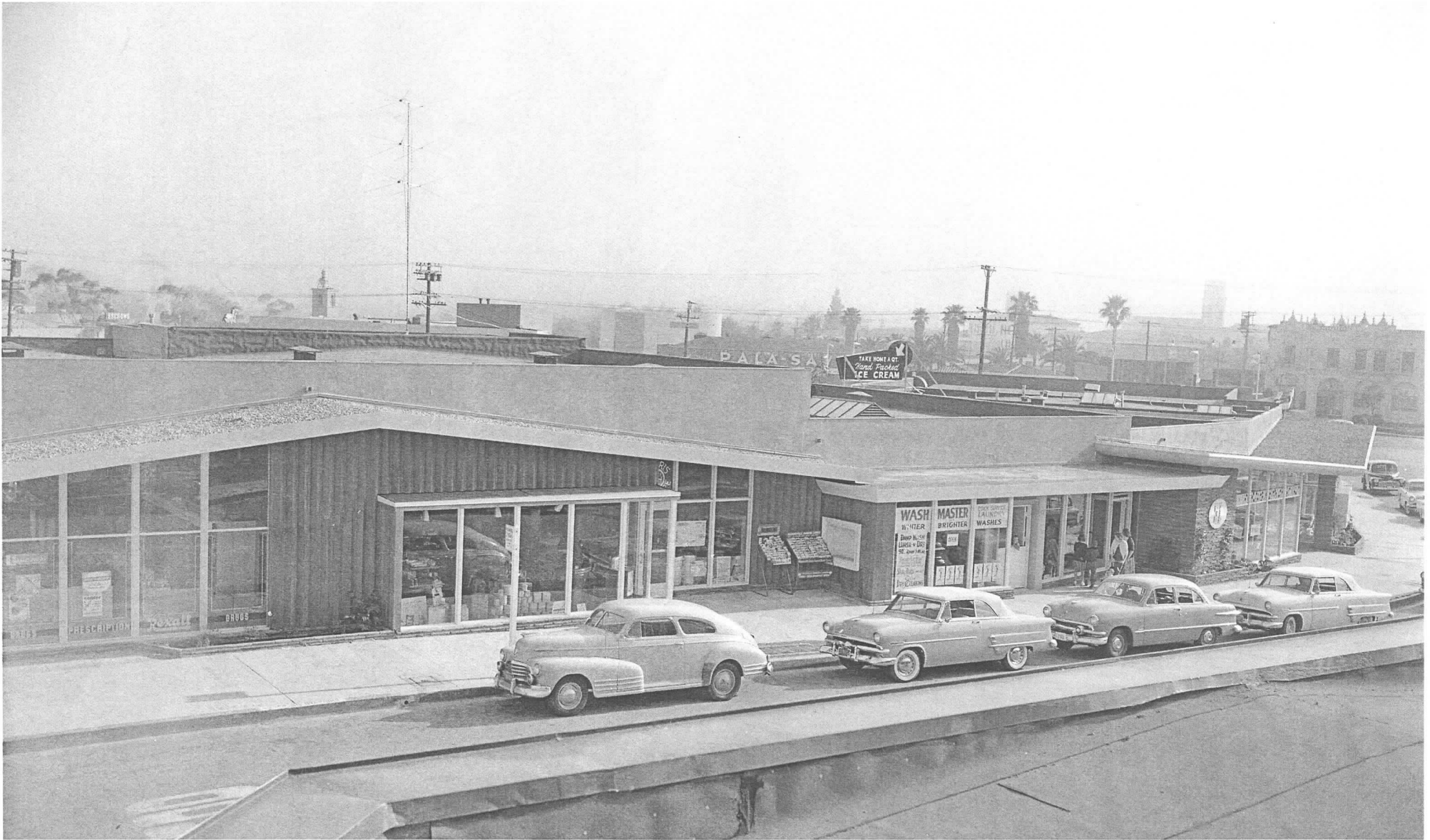
Swarthmore after Completion of East Side April 1954.
