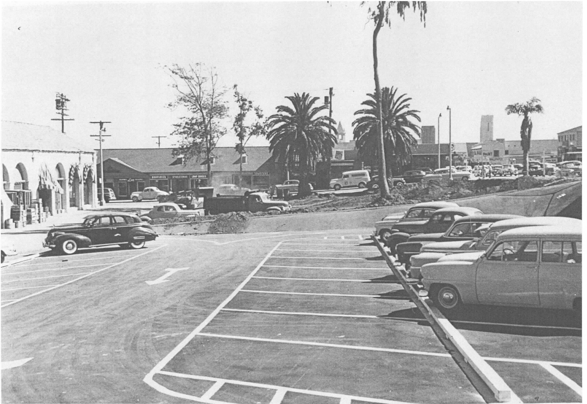
Parking lot and Final Grading for the Medical Building Circa 1958.
