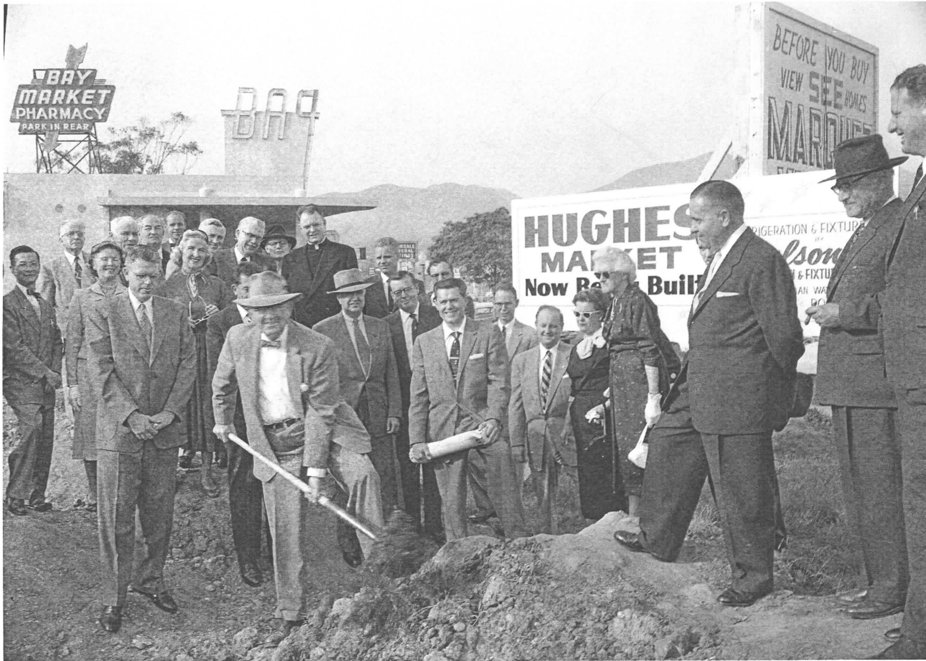
Groundbreaking for Hughes Market January 1956.
